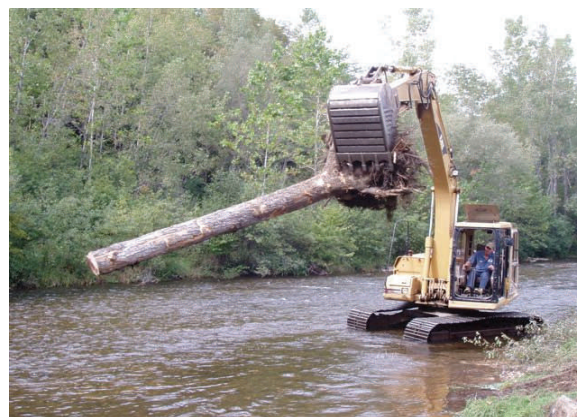
Sand bank stabilization in Manchester.
