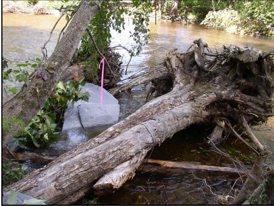
Figure 4. One of 40 artificial structures being constructed in 2006 and 2007 at the Batten Kill Twin Rivers Project in West Arlington, Vermont, designed to create large wood trout cover habitat.
