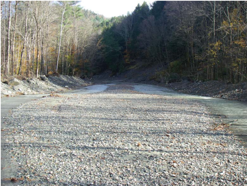
Figure 6. Gilead Brook (Bethel) following extensive streambed and natural wood mining, berming and straightening after Tropical Storm Irene.
