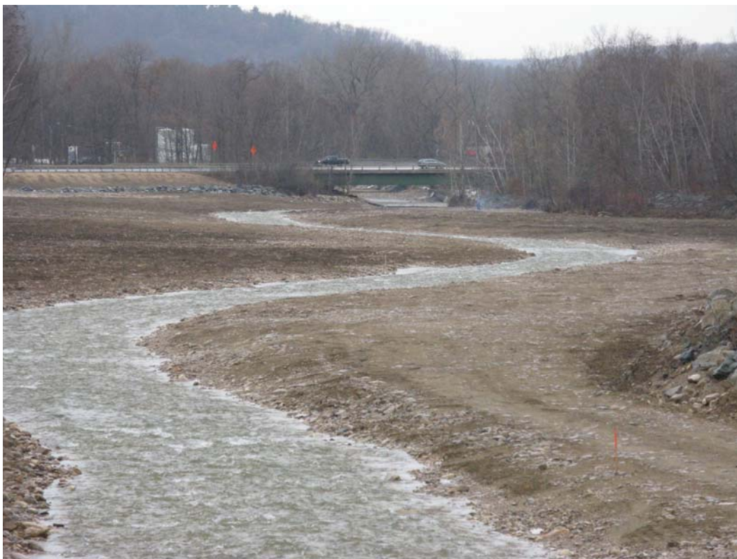
Figure 11. An engineered stream channel of the Roaring Branch (Bennington) provides proper channel and flood plain dimensions, but is devoid of complex aquatic habitat features.
