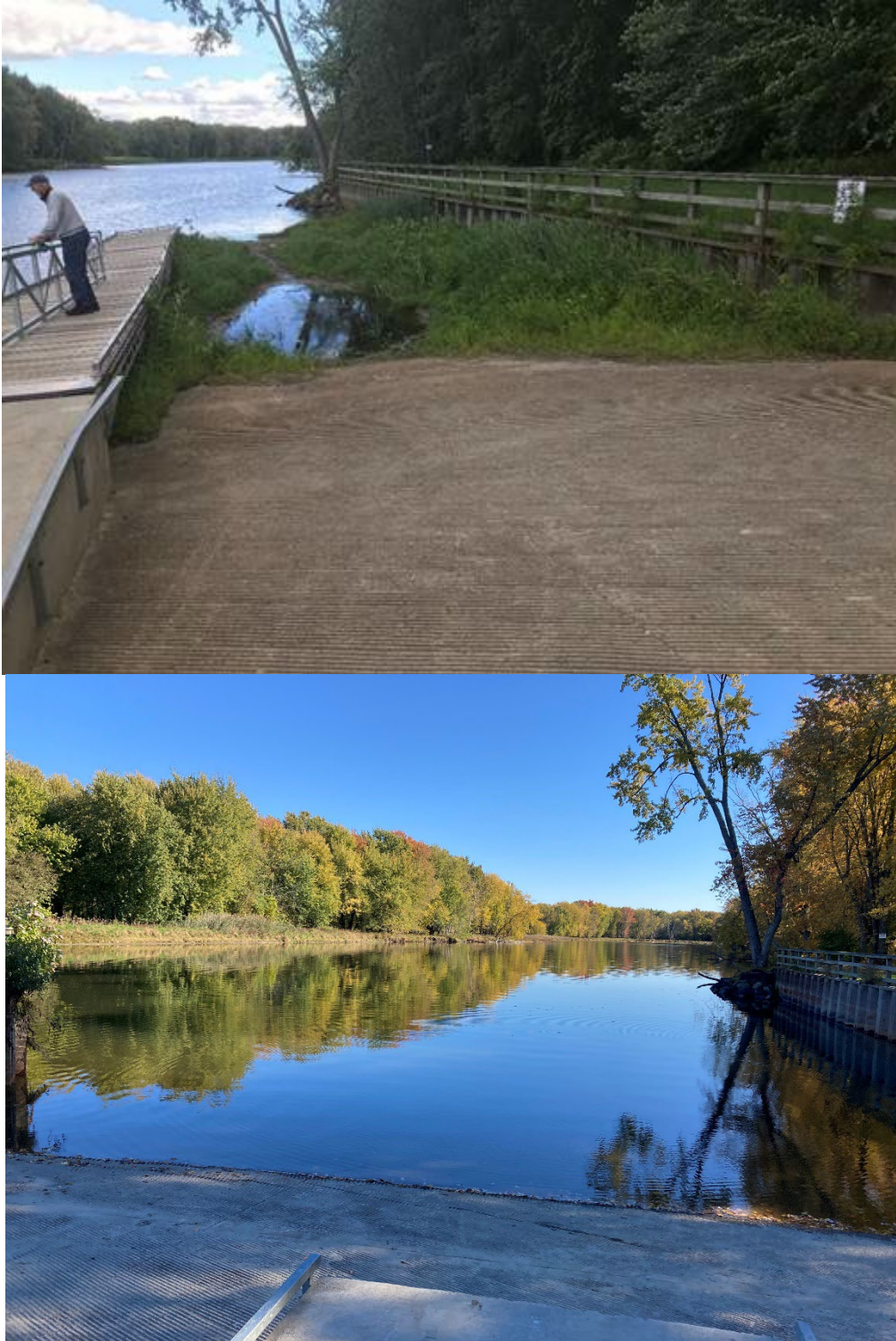
Figure 2. Before and after photos of the Colchester Point Fishing Access Area ramp on the Winooski River in Colchester Point. Severe siltation issues prevented boats from launching during most months of the year. The ramp was dredged this past fall to improve accessibility to the Winooski River and Lake Champlain.
