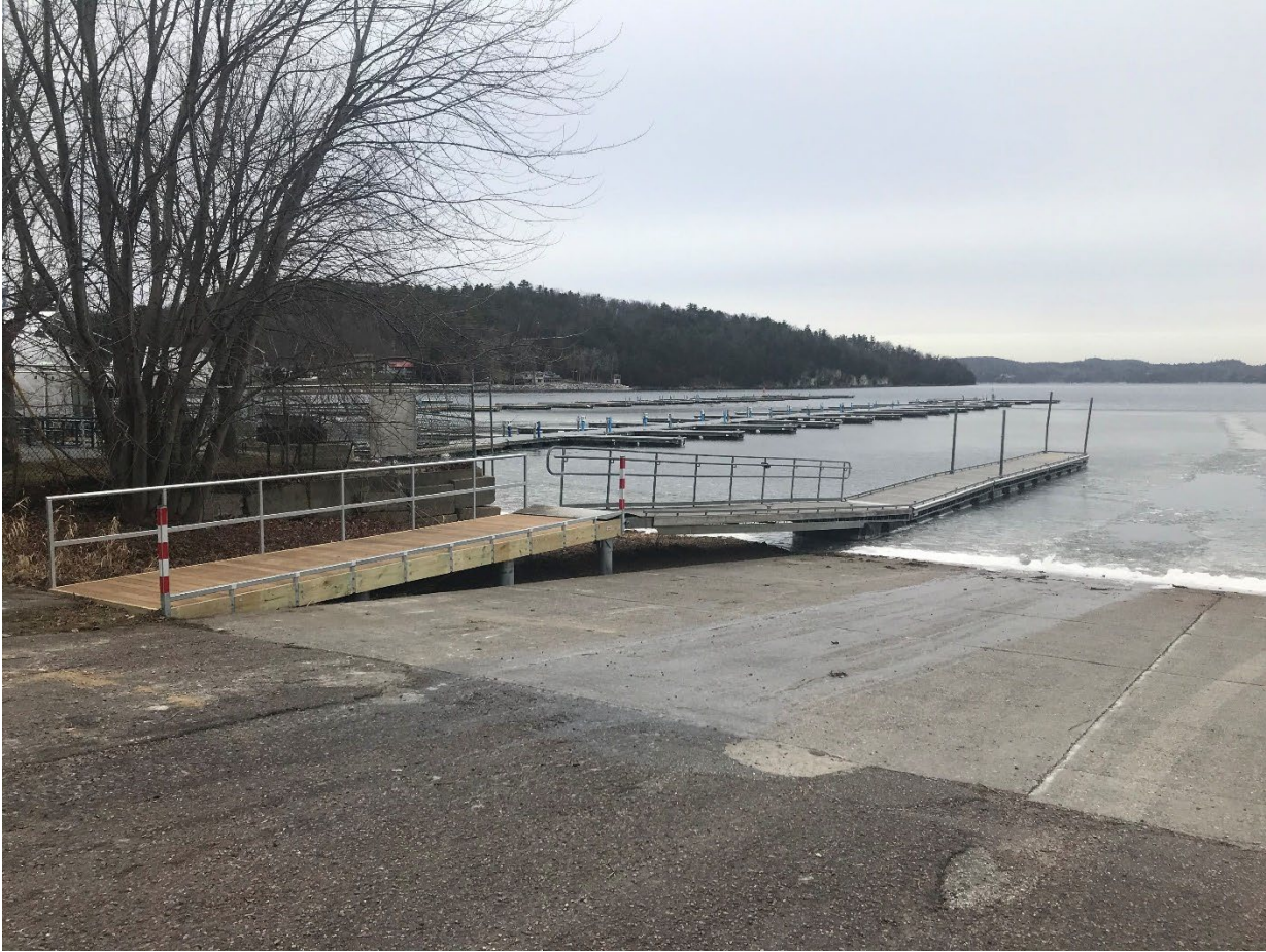
Figure 1. Malletts Bay (Colchester) – New anchoring systems were installed on the two docks in 2020 using CARES Act funding and in 2021 both docks were refurbished by replacing floats, bumpers, and broken planks. This site is the Department’s largest and busiest fishing access area. These modifications will increase the docks’ longevity and boaters’ safety
