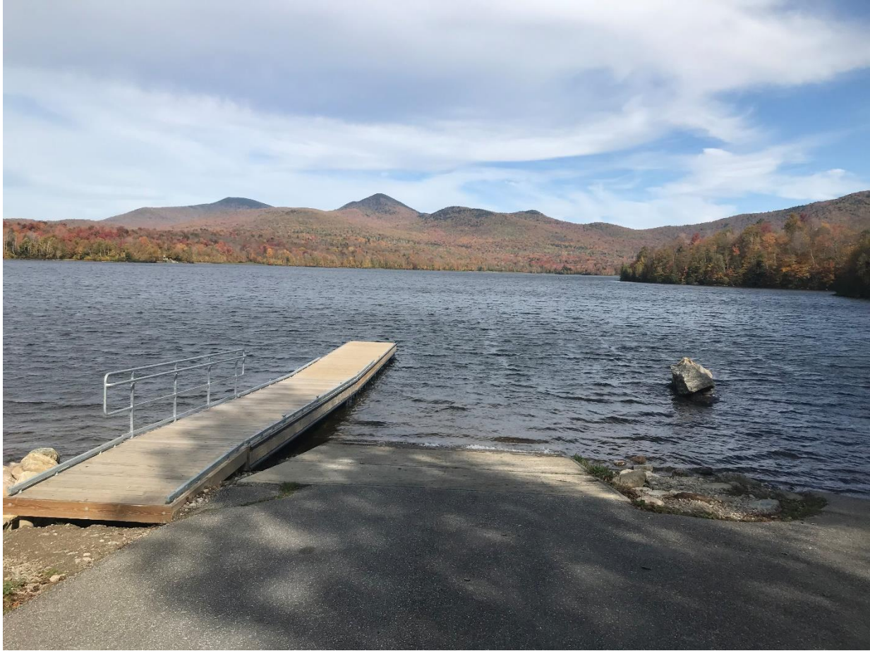
Figure 1. Newly installed 60 ft dock, summer 2019, at the Chittenden Reservoir Access Area in Chittenden, VT.
