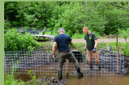
Top: Tyler Brown and Bree Furfey install a beaver baffle. Below: Tyler Brown installs a beaver exclusion fences.
