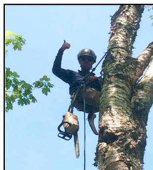
Hazardous tree removal
