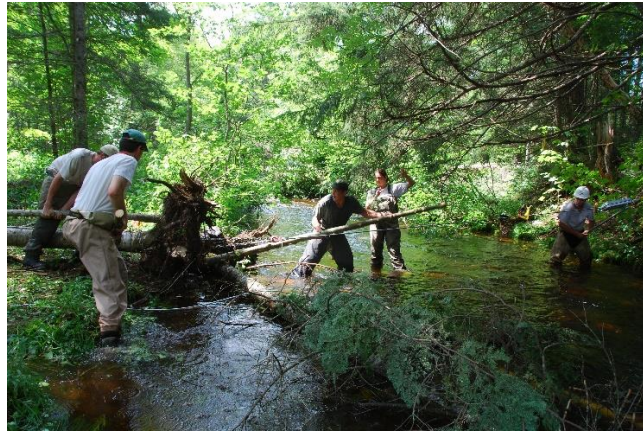
Using the grip hoist to position a tree in the stream.
