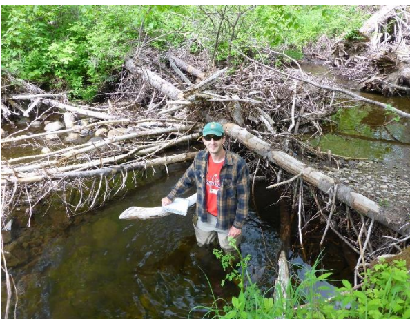
The author standing in a deep plunge pool created by a constructed wood jam.
