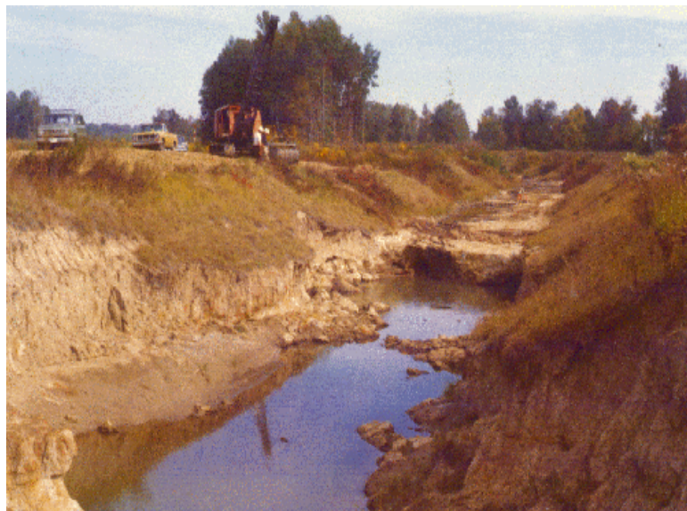
Figure 6. A head cut is a steep drop in the channel bed that migrates upstream.
