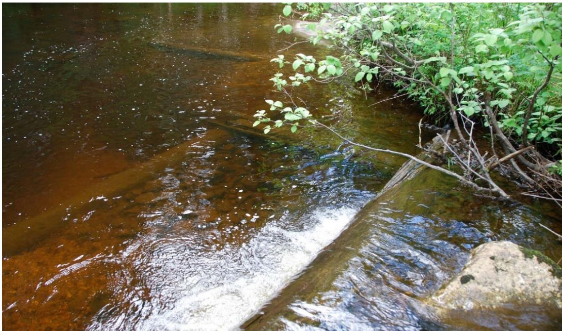
Figure 14. Intact logs at a former log drive dam site. These logs have been here for at least 100 years.
