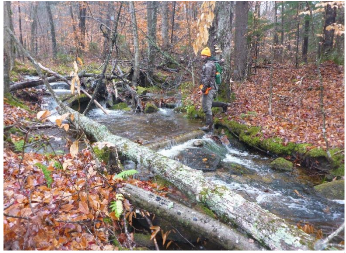
Figure 13. A hand-placed log with a tree felled on top for ballast.
